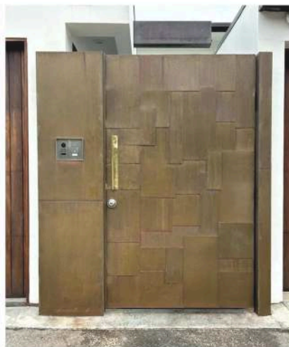
A bronze gate created with carefully welded panels to generate a unique pattern and texture.
