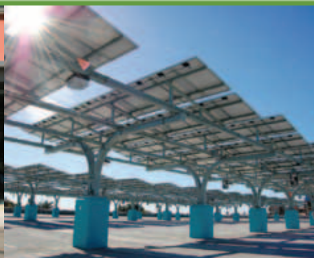
L.A. MISSION COLLEGE'S ROOFTOP SOLAR FARM
