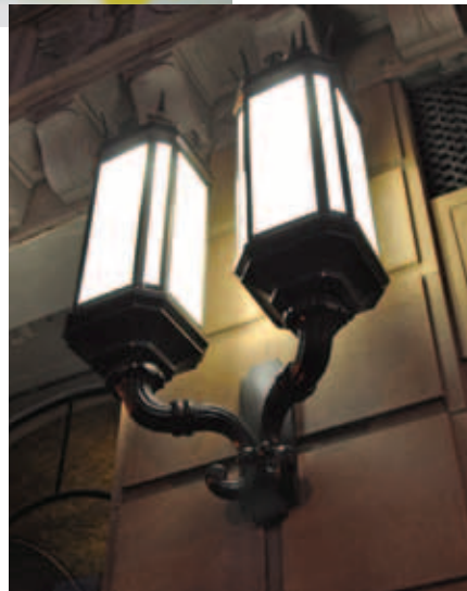
This decorative light by ADG that uses induction technology is installed on the Pershing Square building in downtown Los Angeles.
