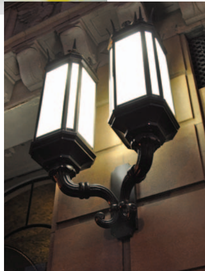
This decorative light by ADG that uses induction technology is installed on the Pershing Square building in downtown Los Angeles.
